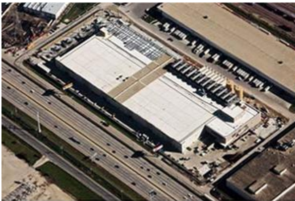
Microsoft's Chicago Data Center October 2008 Photo by McShane Perry Studios, Chicago
